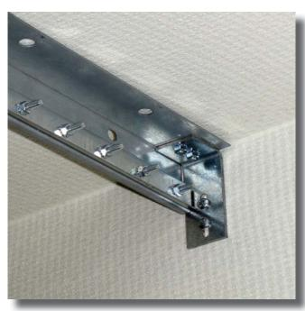
1. Installation of the mounting bar varies depending on type of rear door. With swing doors, the mounting bar can be attached to the ceiling or to the header.
